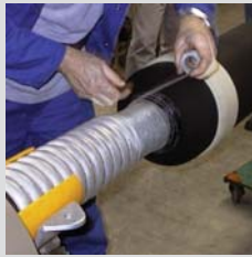
Joint core finishing
