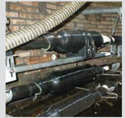
Complete joints in final position
