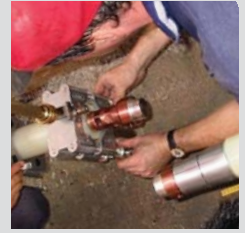
On-site cable end preparation
