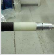
Factory prepared cable end ready for installation
